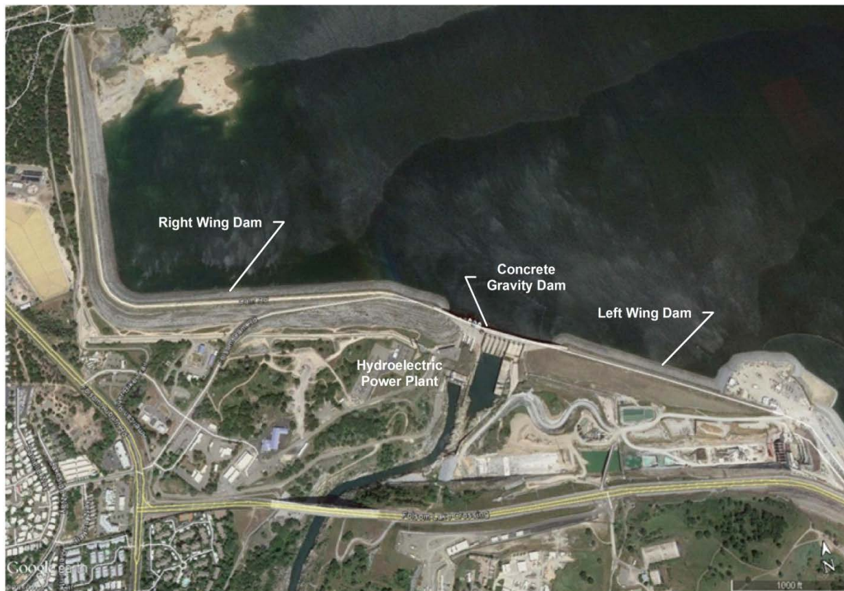
Figure 1-2. Existing Folsom Concrete Gravity Dam and Earthen Wing Dams.
