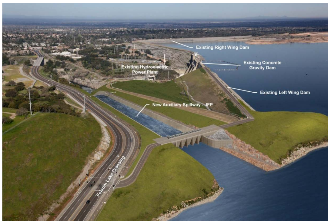
Figure 1-1. Existing Folsom Dam with a Rendering of the New JFP Auxiliary Spillway.
